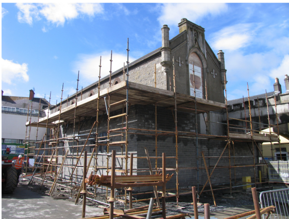
Making Progress: Construction work on new museum extension.
